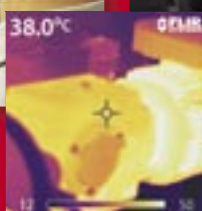
Make quick inspections
