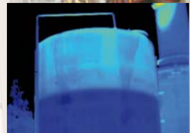
Tank level too low
