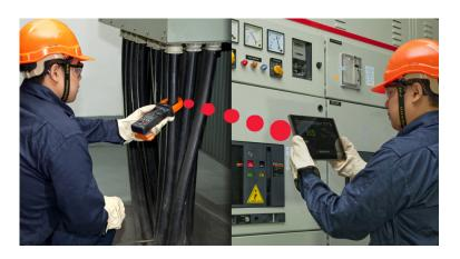
convenient manner. With the U1177A Infrared-to-*Bluetooth* adapter, you can easily monitor measurements and log data up 10-metres range across all Android platform devices—
